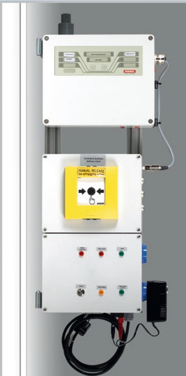
The fire extinguishing system consists of an infrared fire and smoke sensor, a detector electronic housing, it's own UPS box with charging unit and backup battery, an electromechanical trigger device and a bottle with Argon or Nitrogen.
